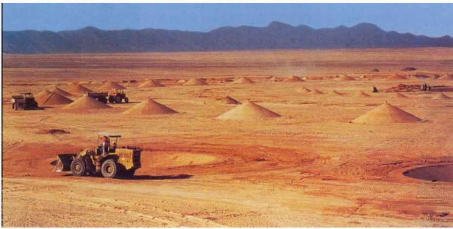
Left While constructing the double spiral cones, the D.A.ST. team found that the positive and negative cones had to be dug in height and depth sequence: from the largest to the smallest.
